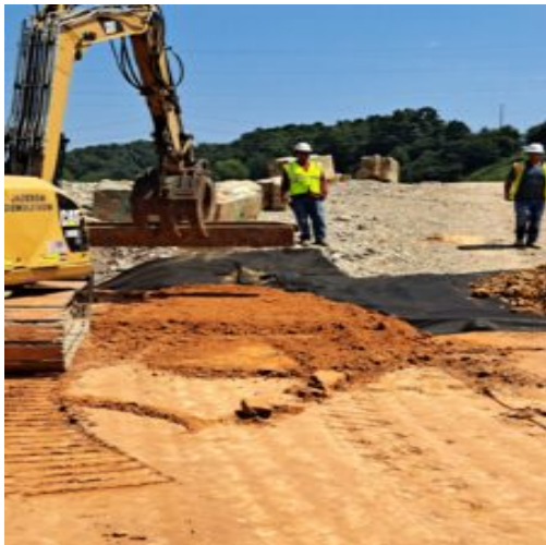
Covering the geo-fabric with fill-material
