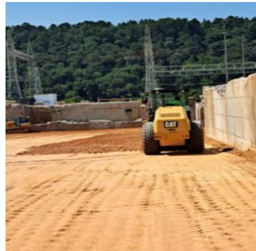
Vibratory roller for compaction of fill material in section 2
