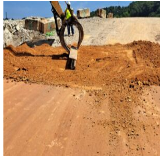
Spreading and covering the fill-material on the geo-fabric on the ramp of the basement
