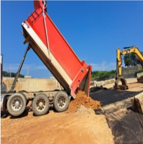
Placement of the fill material on the ramp
