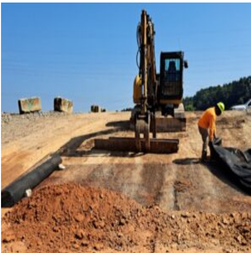
Placement of the fill material on the ramp
