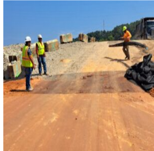
Placing geo-grid
