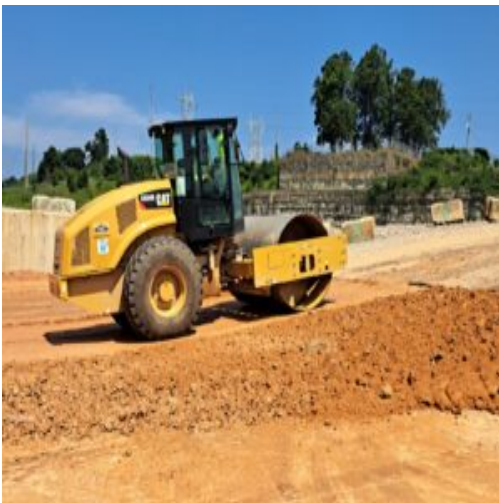
Compacting fill-material using vibratory roller
