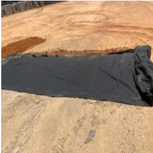
Placed Geo-fabric after the placement of geo-grid
