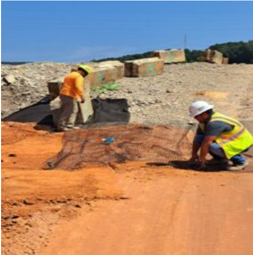
placement of the geo-grid at the bottom of the ramp
