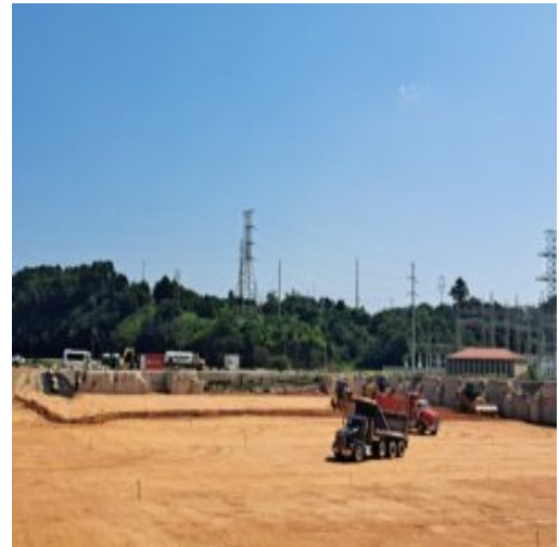
Placed the fill material in mid way of the section 1 basement area B7
