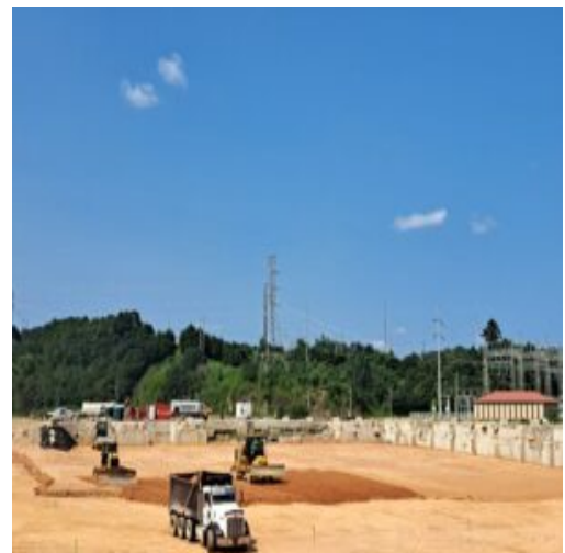
Fill materials placed in Section 1 basement area B7
