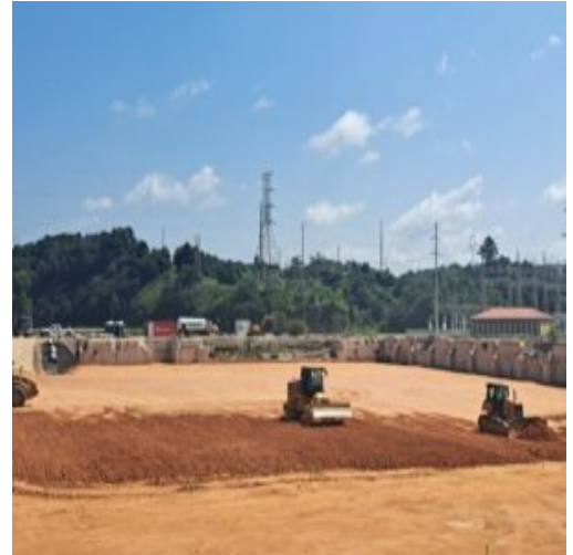
Placed the fill material in section 2 part 1
