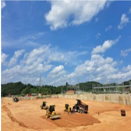
Placed the fill material in section 2 part 1
