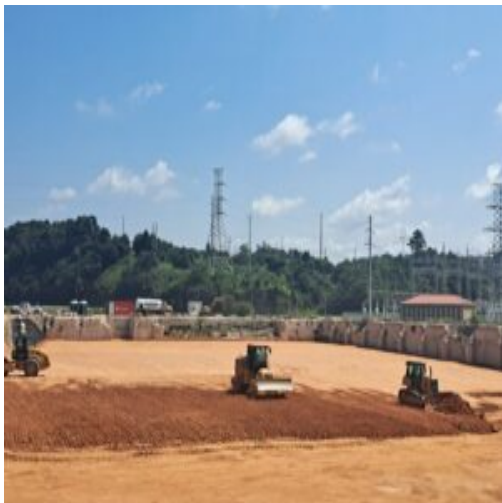
Placed the fill material in section 2 part 1
