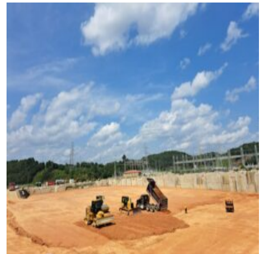
Placed the fill material in section 2 part 1
