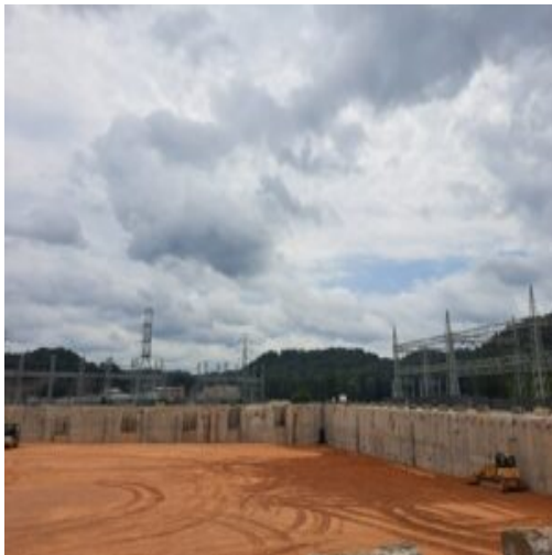
The fill materials placed in section basement area G7
