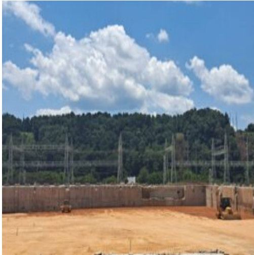
Placement of fill material section 2 part 2
