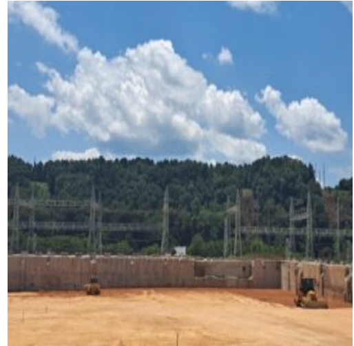
Placement of fill material section 2 part 2
