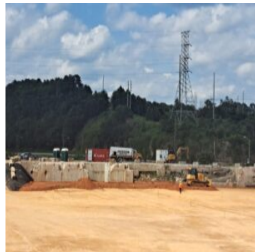
Started the placement of fill material in section 1 basement area B7
