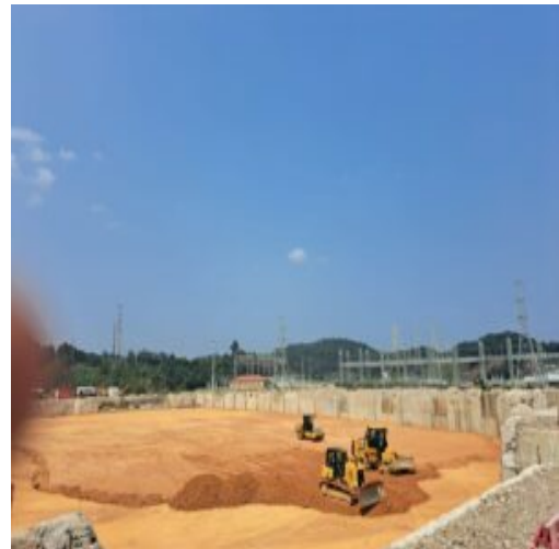
Placement of fill material in section 2 part 1
