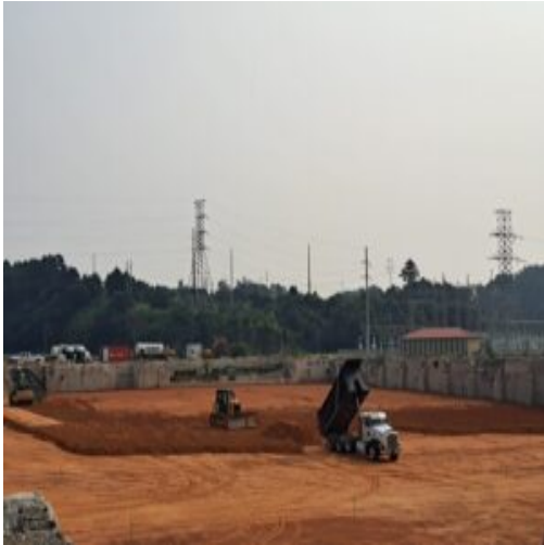
Started the placement of fill material in section 2
