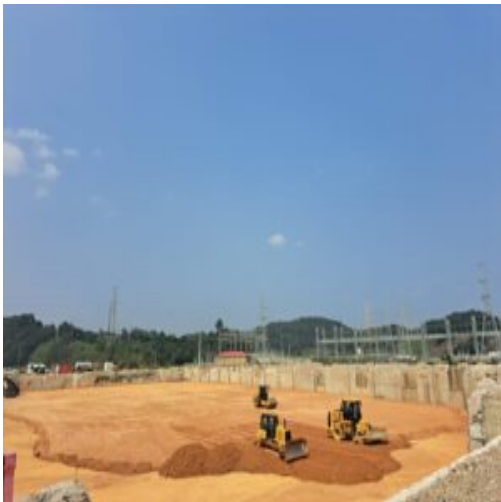
Placement of fill material in section 2 part 1
