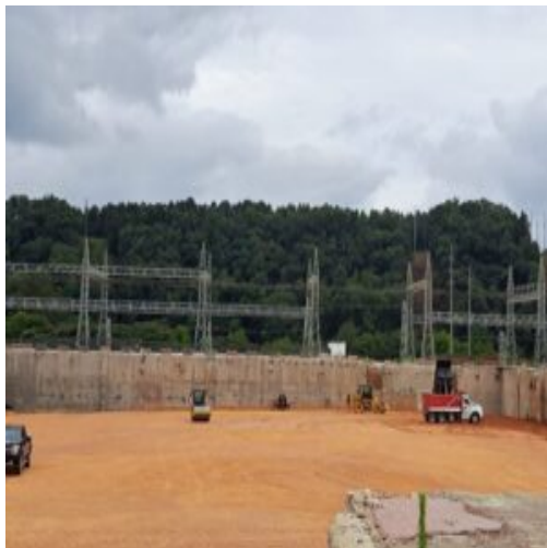
Placement of fill material in section 2 basement area G7
