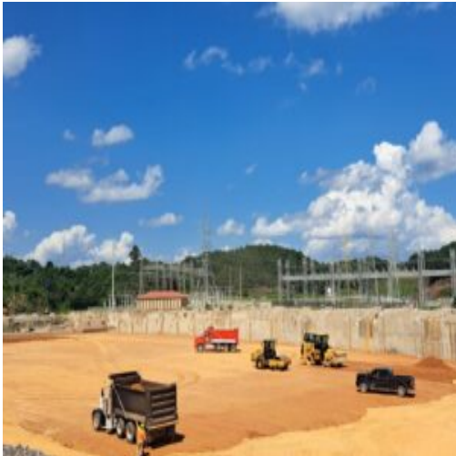
Placement of Fill material in Section 2
