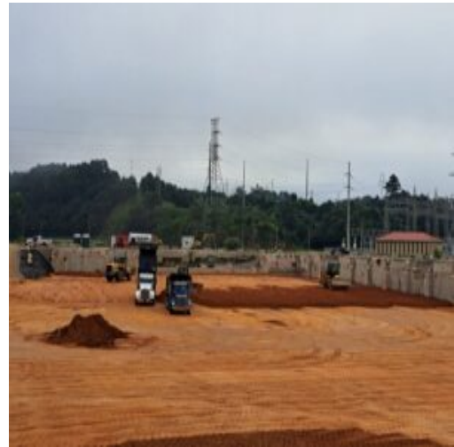
Continued to place the lift in section 2 of the basement
