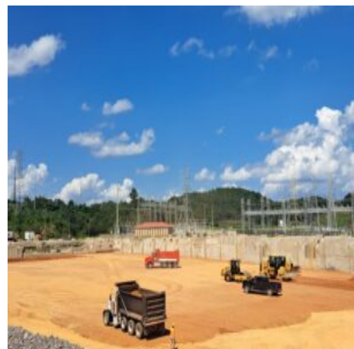
Placement of Fill material in Section 2
