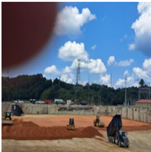
Fill material continued to Section 2
