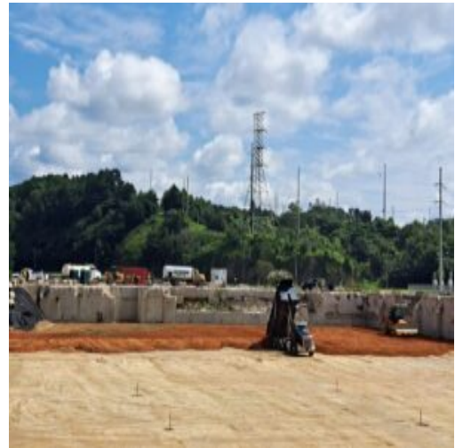
Placement of Fill material in section 1 basement are B7
