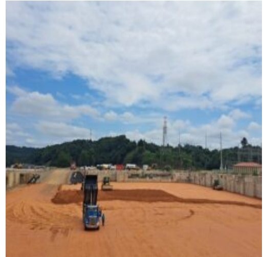
Fill materials were placed and compacted in section 1 basement area B7
