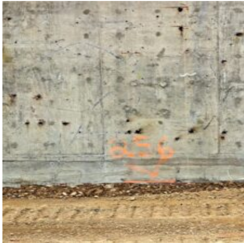
Elevation of the test location
