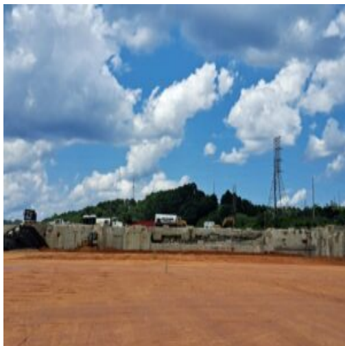
Started the placement of new lift placement in section 1 basement area B7
