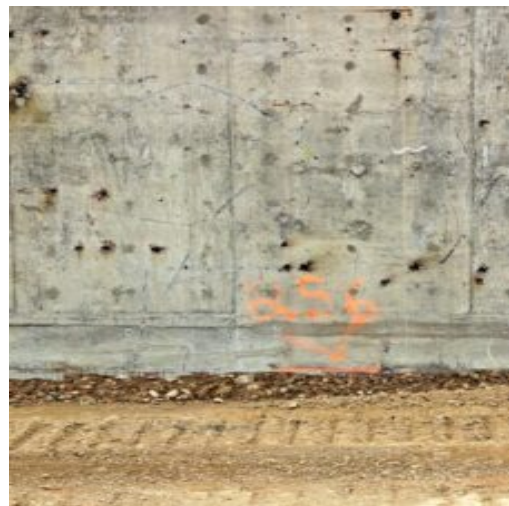
Elevation of the test location
