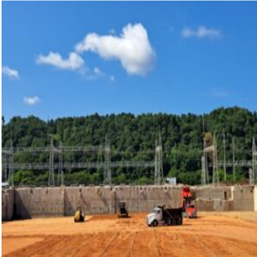
Placement of fill material in the section part 2 in the basement.
