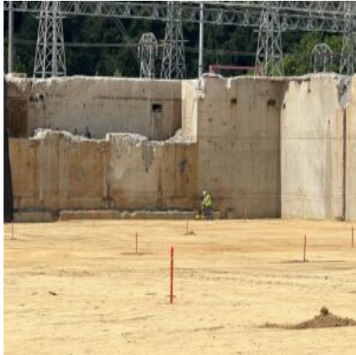
Plate tamper compacting the material along the wall.
