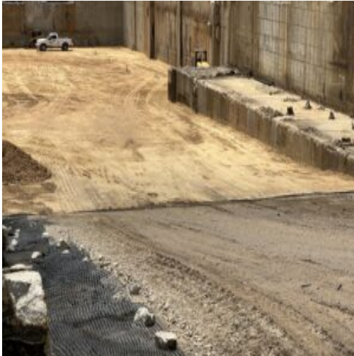
Backfill being placed as lift 8 in the Section 2 area
