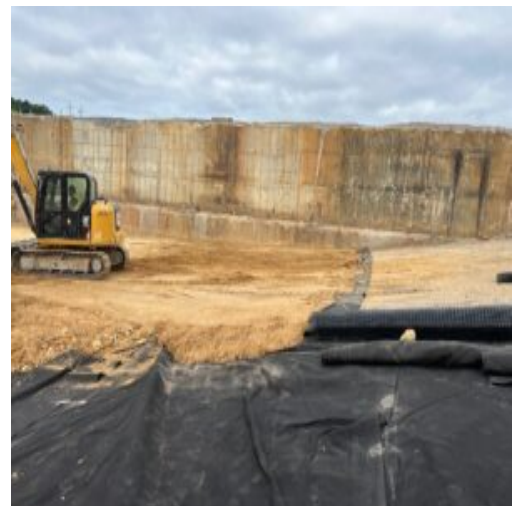
Geotextile and Geogrid as being installed
