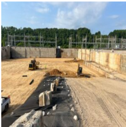
Geotextile and Geogrid as being installed
