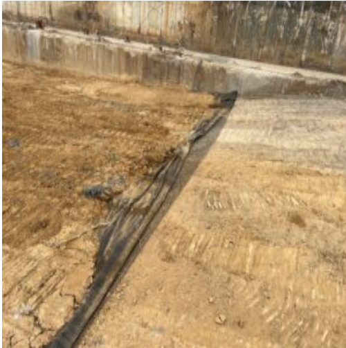
Geotextile and Geogrid as being installed
