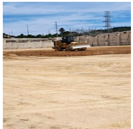
Compaction using the roller and dozer.
