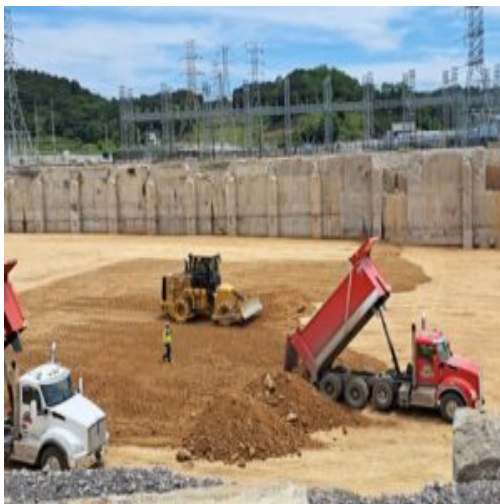
Loads received and delivered to the site for the placement in section-1.
