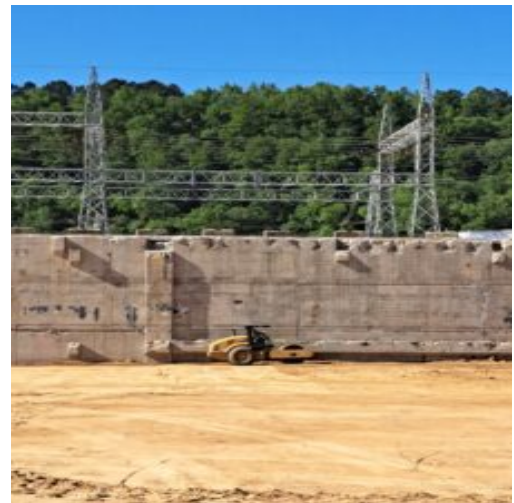
compaction using the roller in section-2 south end wall side.
