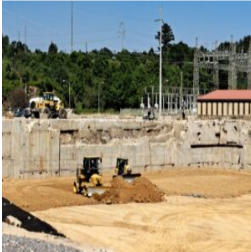
Placement of lift-10 in section-1 basement area B7.
