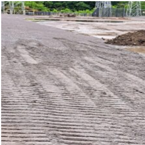
Placement of 825-B crushed stone beside the west wall of the top of the basement.
