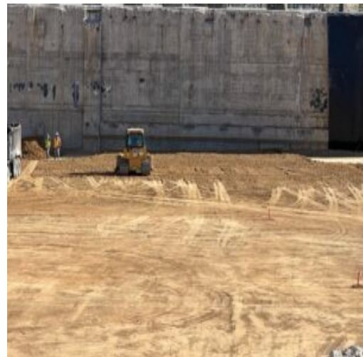
Compaction efforts in Section 2
