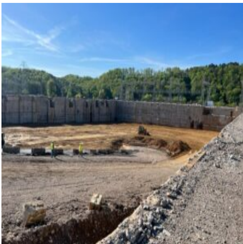
Grading operations - spreading fill material and exposing it to facilitate drying.
