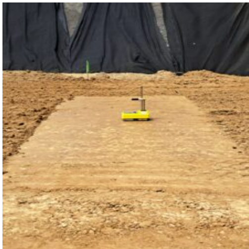
Nuclear Gauge test was Performed in basement section-1 area B7
