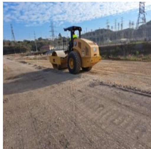
Area H6 being compacted
