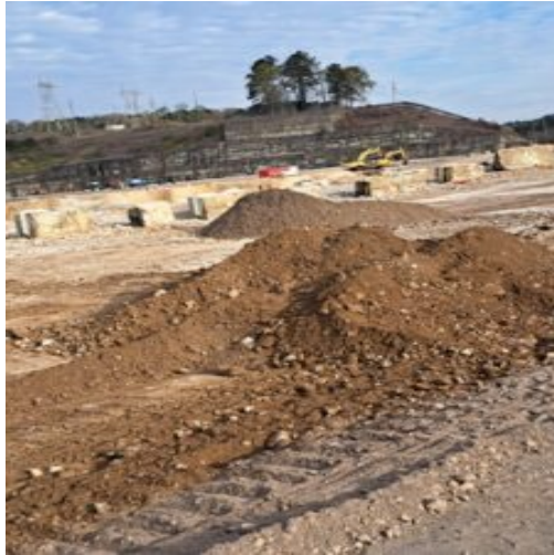
Crushed concrete being placed near the inlet in H6
