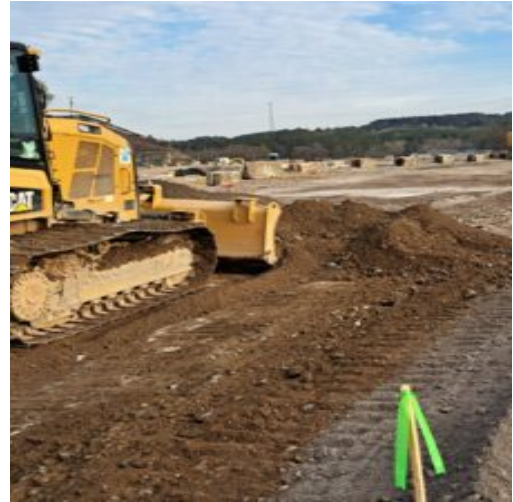
Crushed concrete being placed
