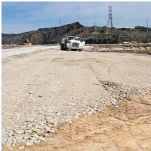
Water truck conducting proof roll in area H6
