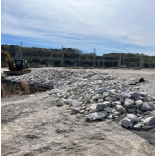
Riprap placed in section H6
