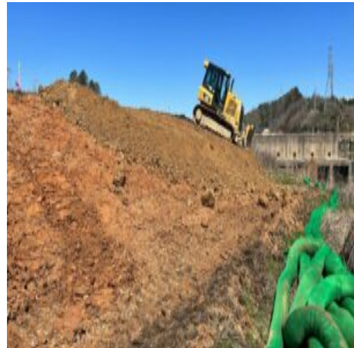
The slope being constructed in section F6
