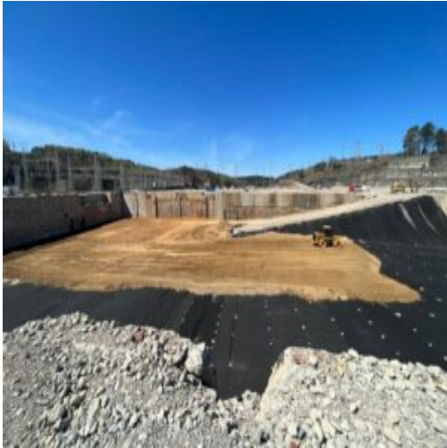
Fill is being placed in the basement as seen from the top of the east wall.
