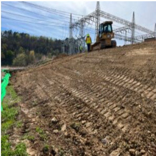
Slope construction at 1400 hrs
