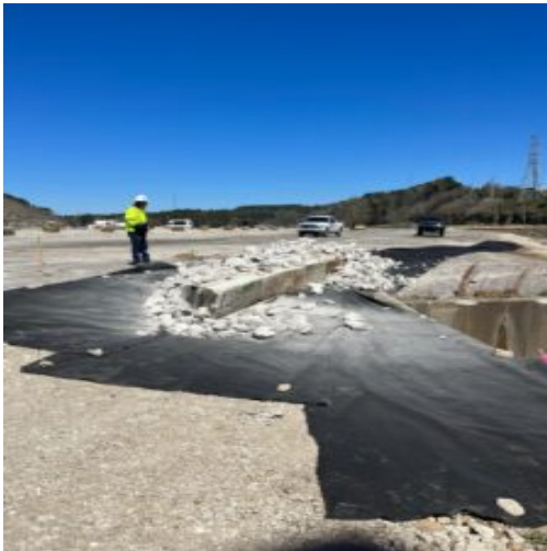
Concrete blocks placed in H6
