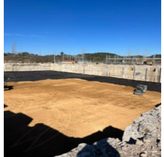
Placement of Fill material and compacted using CAT 815 in the basement.
