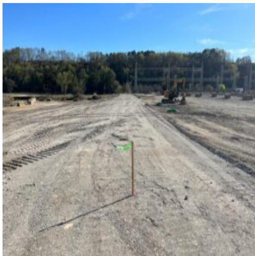
825B Place and compacted
