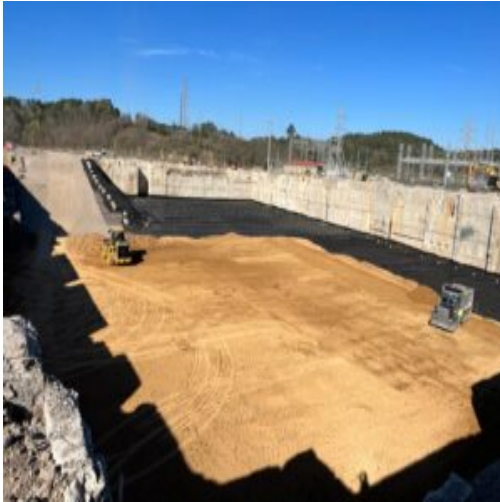
Placement of Fill material and compacted using CAT 815 in the basement.
