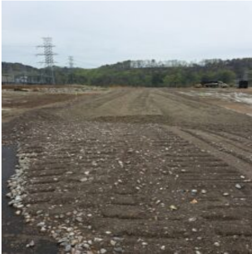
825B Placement 8" loose lift facing south.
