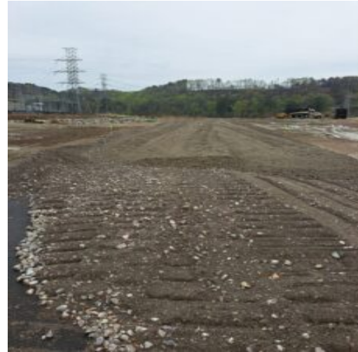
825B Placement 8" loose lift facing south.
