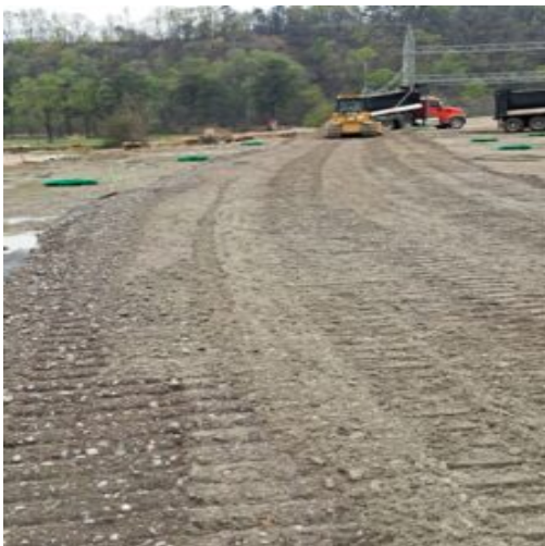
825B Placement 8" loose lift facing south.
