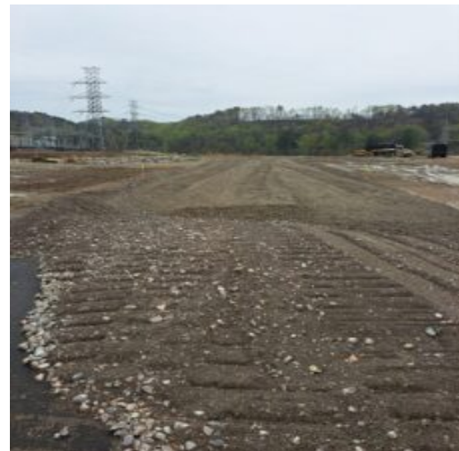
825B Placement 8" loose lift facing south.
