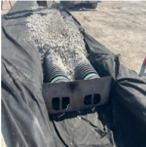
Steel plates cover pipe opening in the north trench. Four 5" - 6" holes were cut in steel to facilitate water flow and prevent rip rap from migrating into drains.
