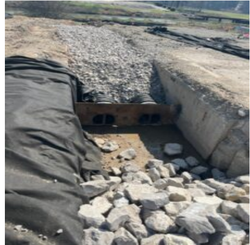
Steel plates cover the pipe opening in the south trench. Four 5" - 6" holes were cut in steel to facilitate water flow and prevent rip rap from migrating into drains.
