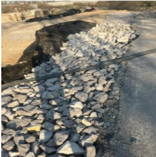
Steel plates between pipe and rip rap in south trench
