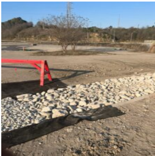
Steel plates between pipe and rip rap in north trench
