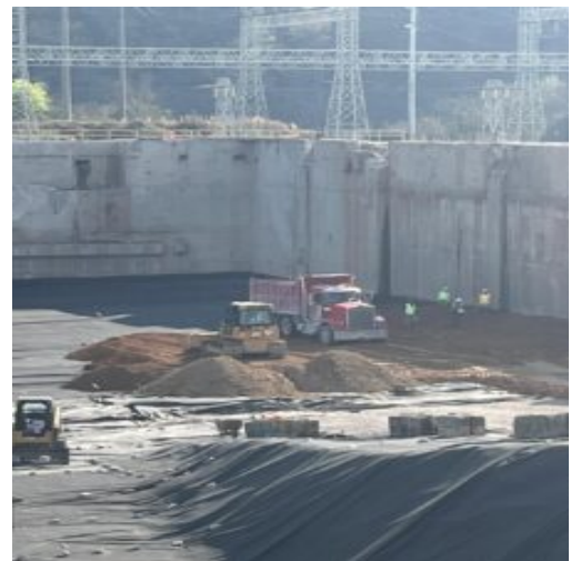
Clay being placed
