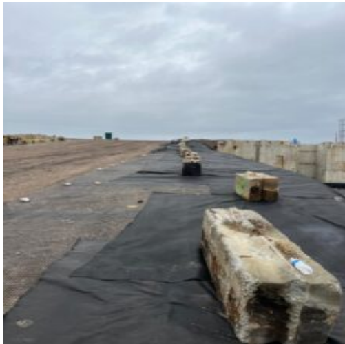
Terrafabric in the basement's upper half on the ramp's east slope
