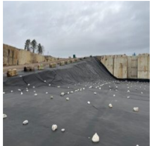
Terrafabric in the basement's upper half on the ramp's east slope
