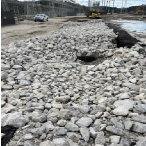
Rip-rap installed in the trench in areas F7 and F8
