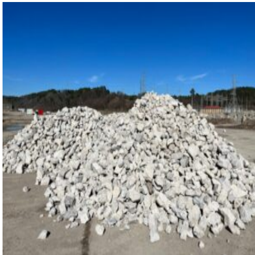
Riprap delivered and staged new the south east corner of the basement. Area G6
