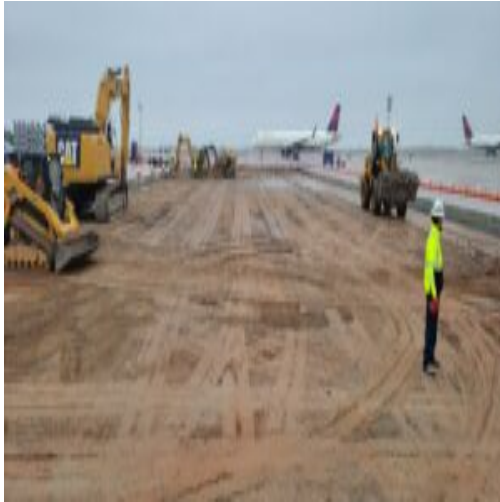
Proofroll within Phase 1 of the project
