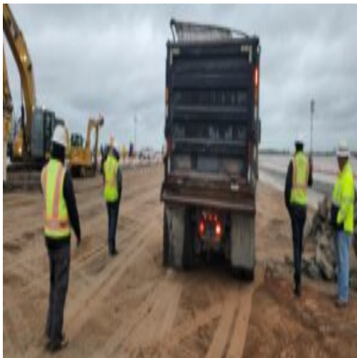
Proofroll within Phase 1 of the project
