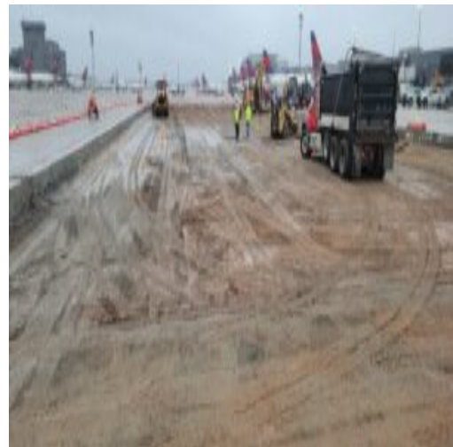
Proofroll within Phase 1 of the project
