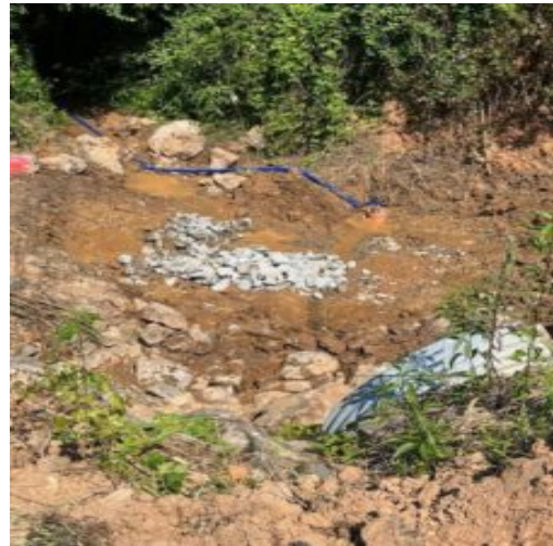
Rip rap placement in remediated zone
