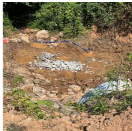
Rip Rap placement
