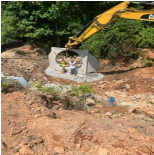
Placement of headwall
