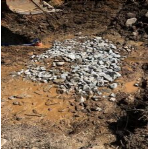
Lift 2 of riprap placed
