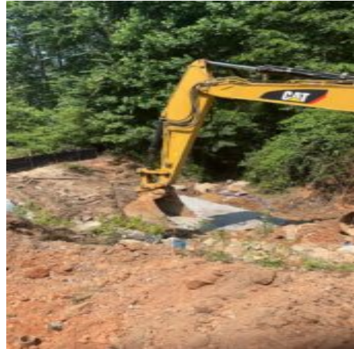
57 stone placement atop rip rap
