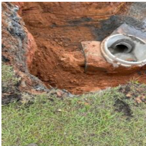
high moisture soil removed at A4
