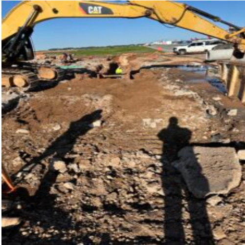
Excavation/placement storm drain pipe
