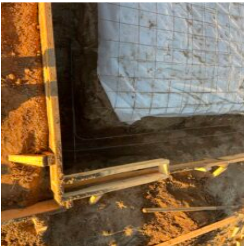
After pultes foundation team dug out the soft spot.
