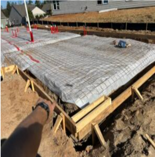
Area that required remediation on lot 62-14
