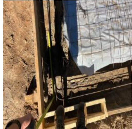
3 feet in length each direction and 2 feet deep.
