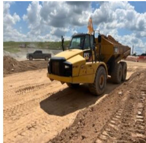
Proofroll within taxiway station 409+00 to 408+00
