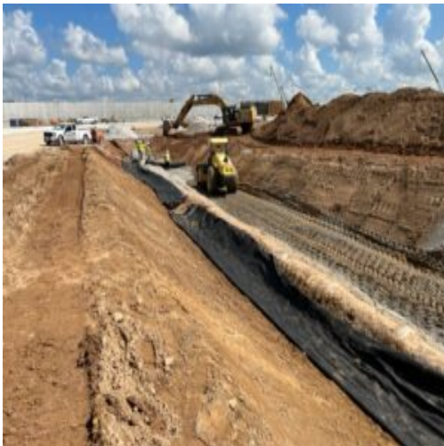
I3 and I4 structures. backfilled with M10 sand after installing fabric.
