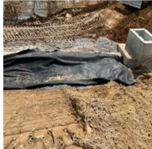
#57 stone placed and covered with fabric between I3 and I4 structures.
